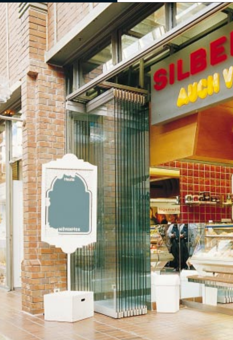
Stacking tracks for panels arranged parallel to the shopfront
